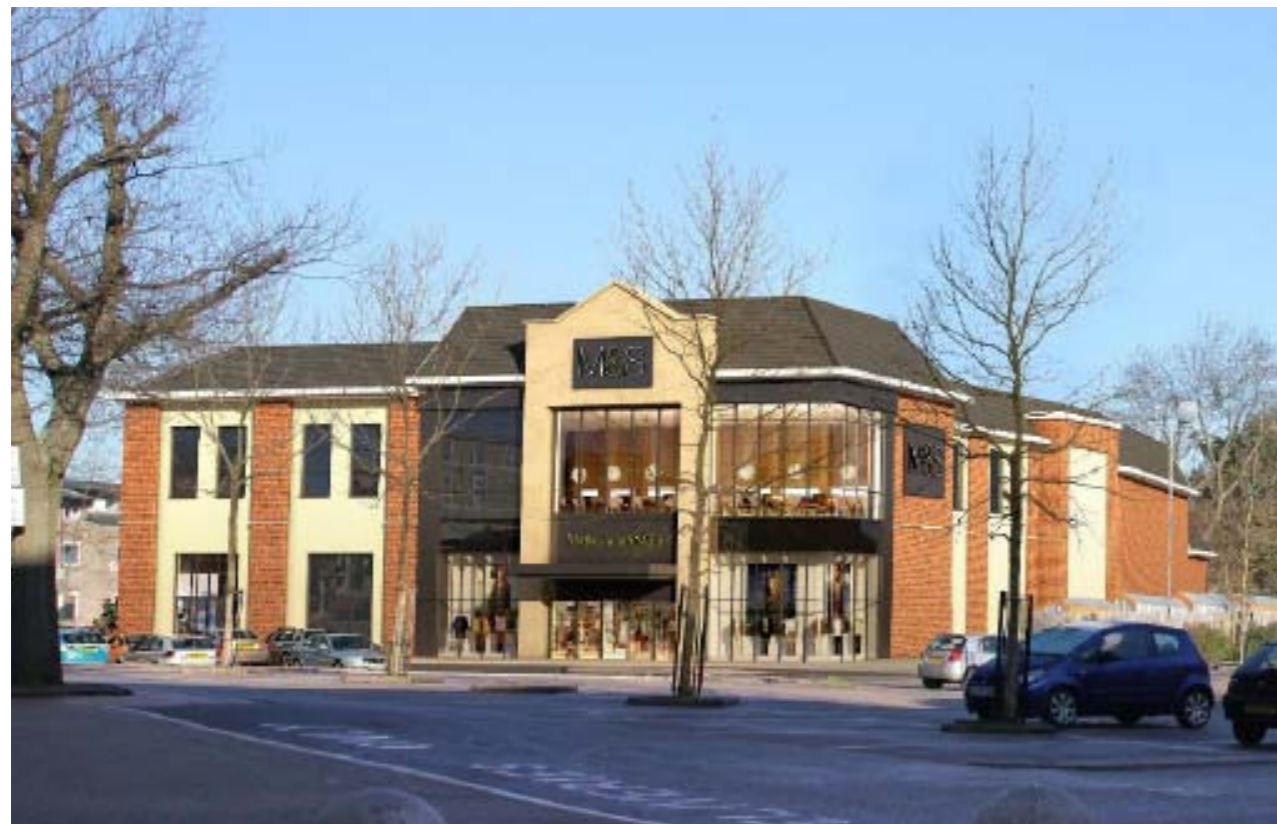
Sevenoaks Blighs III town centre mixed use redevelopment by Reef Ltd where Chase & Partners advised Sevenoaks District Council on all aspects of the proposal including land sales to the promoter.
