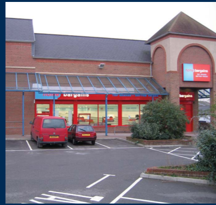
Northampton: St Peters Way Retail Park Rent reviews and Asset management for ING Real Estate Investment Management. Surrender of Aldi lease and new letting to Home Bargains who opened 1st November 2004.
