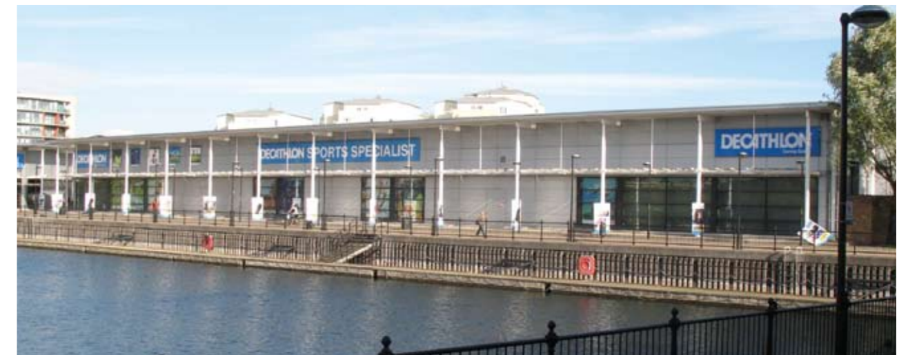
Southwark - 2010 - Rent review of Decathlon units, Canada Water, on behalf of Conrad Phoenix Properties
